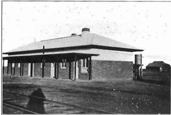
FIG. 4.—REPEATER STATION BUILDING: TRANSCONTINENTAL ROUTE.
