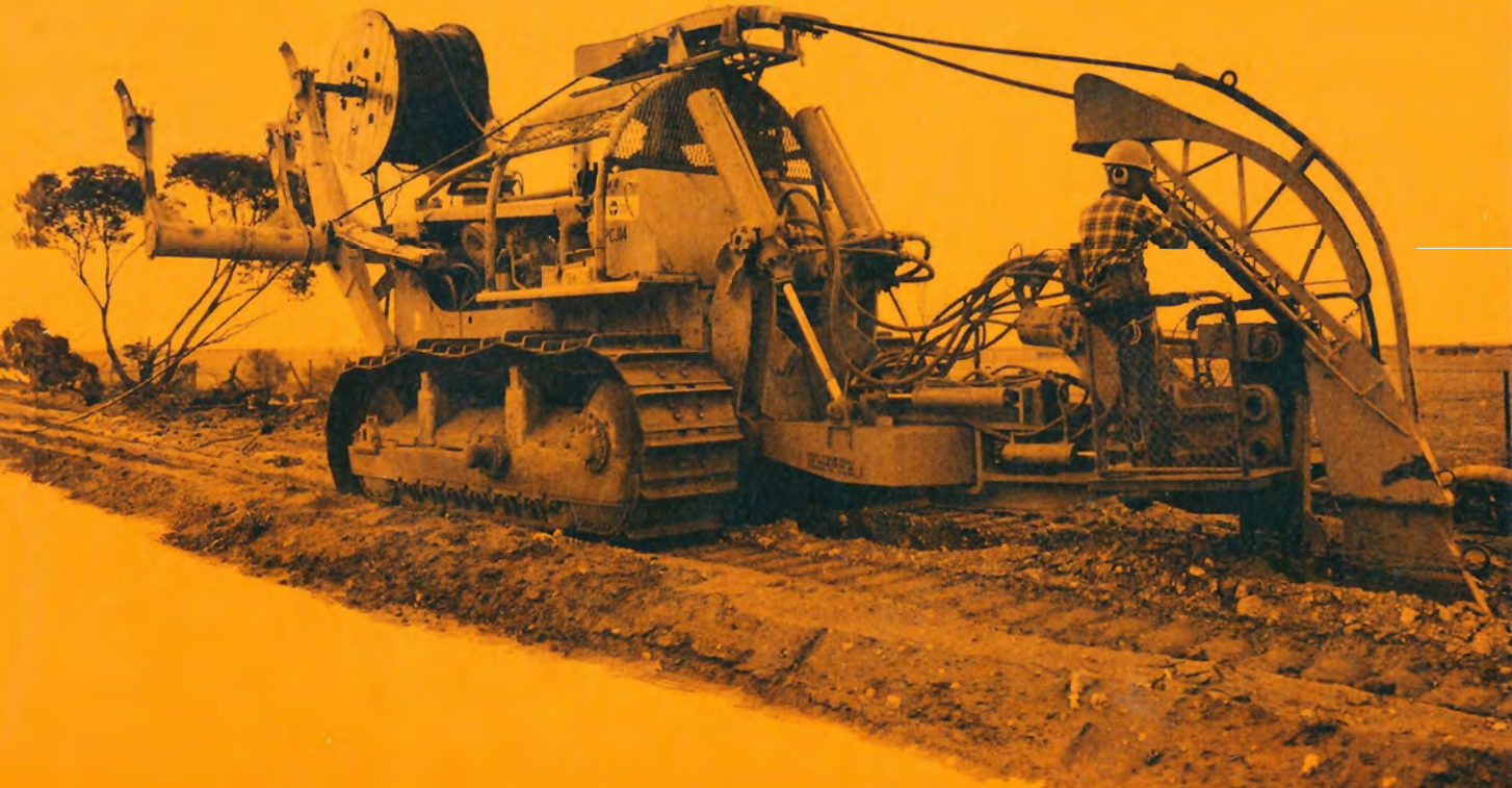
Modern coaxial cable laying machine.
