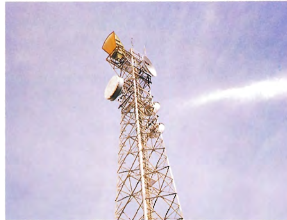
Top section of the tower
