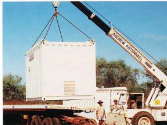
Unloading battery shelter.
