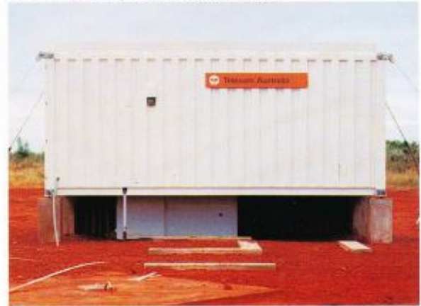
Shelter in position.
