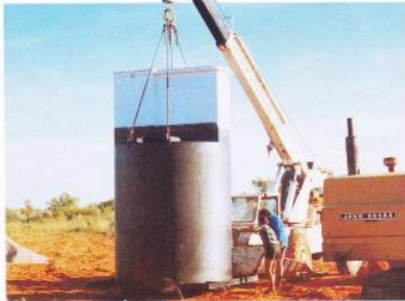
Equipment container being lowered into position.
