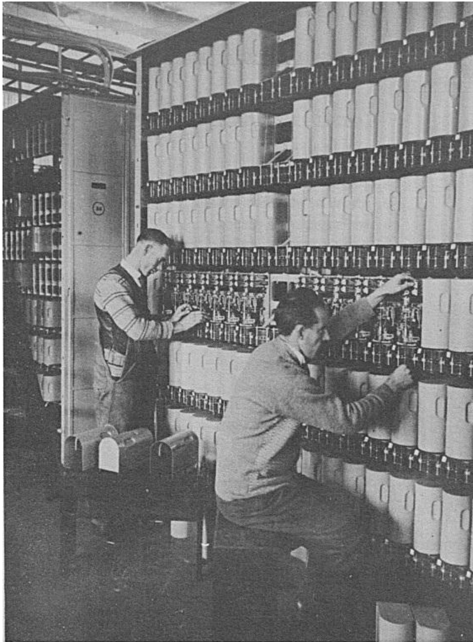
TECHNICIANS MAKING FINAL ADJUSTMENTS TO SELECTORS IN AN AUTOMATIC EXCHANGE PRIOR TO THE "CUT-OVER".
